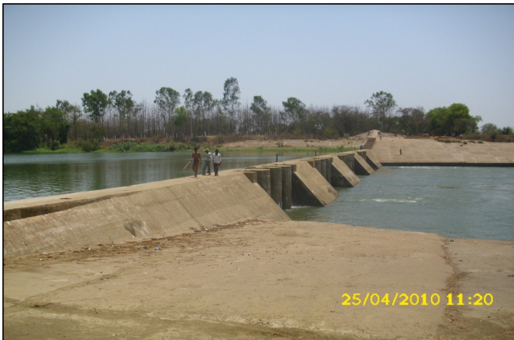
Bhatagaon anicut providing water supply to Raipur city
