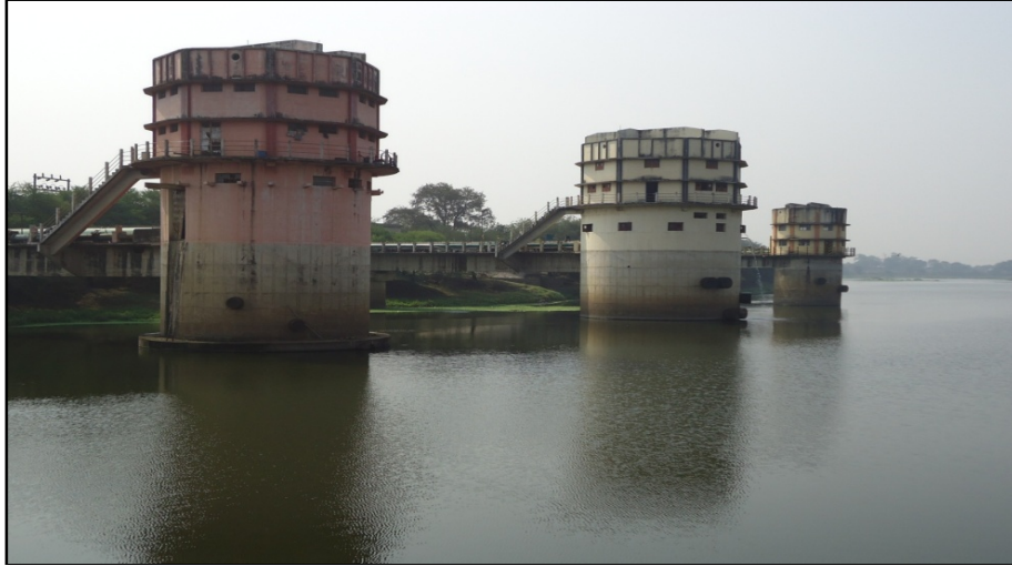
Pump house at Murethi anicut providing water supply to Silthara industrial area
